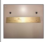
Unless Mounting into a stud, drill two 5/8" diameter holes that match the distance of the two holes in the Cleat(B) when it is in the desired position on wall. These holes will be used to mount the cleat.
