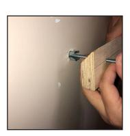
With the wings screwed on, insert the bolts into the holes drilled in Step 2. Pinch the wings and insert them into the holes. Push Bolt into hole until wing opens on other side of drywall.
